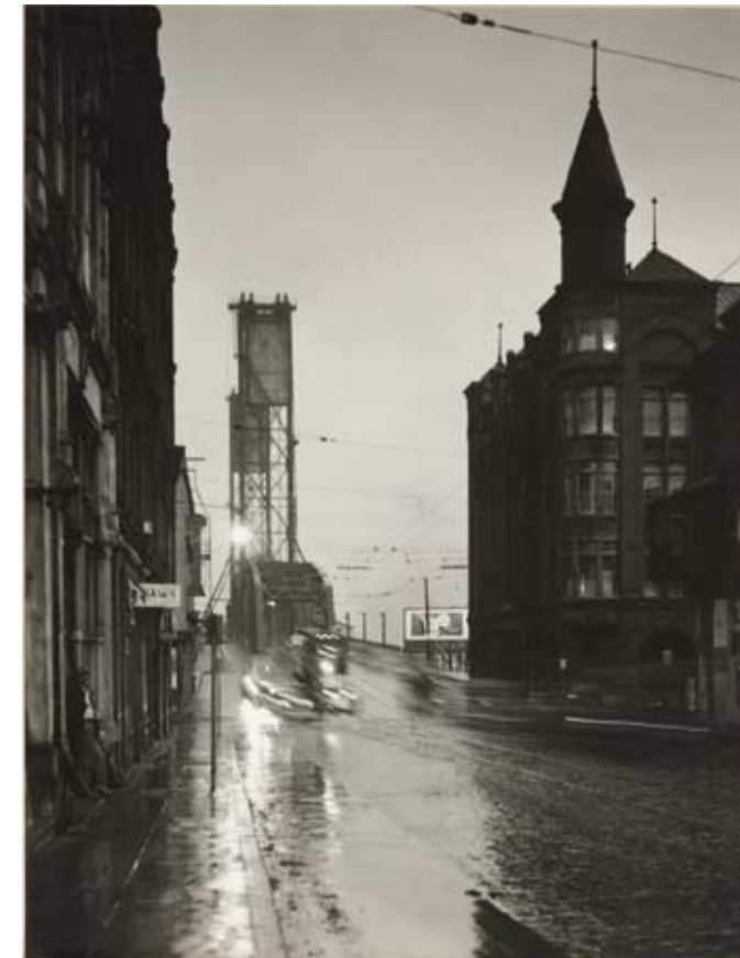
Figure 6. Minor White. Bridge (Morrison Street?) , Portland, 1939. 11 x 8.5 cm. MWA 39–550.
